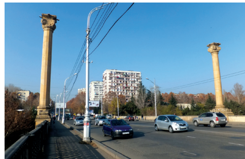
Didube bridge in Tbilisi
