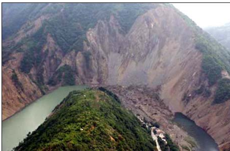
Fig. 1. View of the earth-fill dam blocked up and destroyed as a result of an earthquake in China
