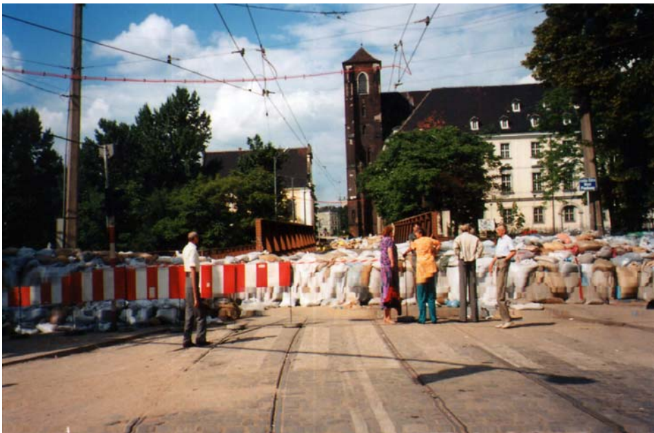
Photo 1. Piaskowy bridge, flood of July 1997
