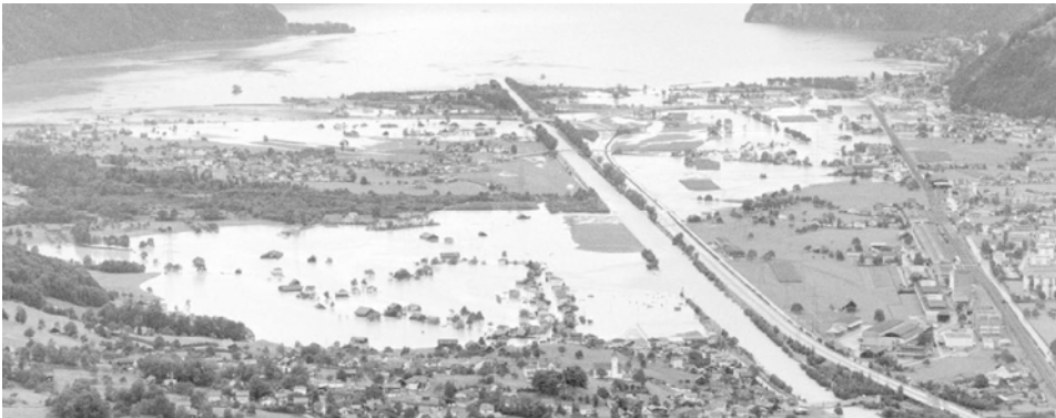
Fig. 1. Dam ruptures in the valley of the Reuss, august 1987
