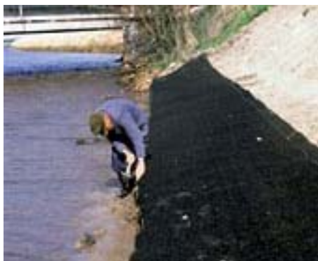
Photo 4. Insuring the stability of river bank by means of "Sekumat"
