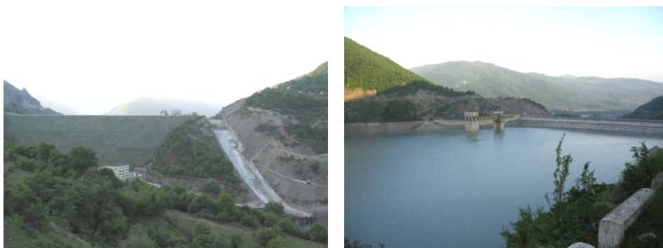
Fig. 2. General view of the headrace and tailrace of the Zhinvali Earth Dam
