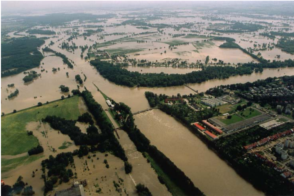
Photo 4. Bartoszowice weir, flood of July 1997
