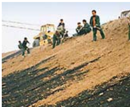
Photo 5. Process of mounting "Sekumat"
