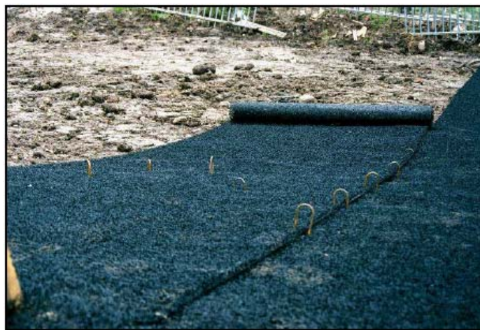
Photo 8. Process of spreading and fastening of “Sekumat”
