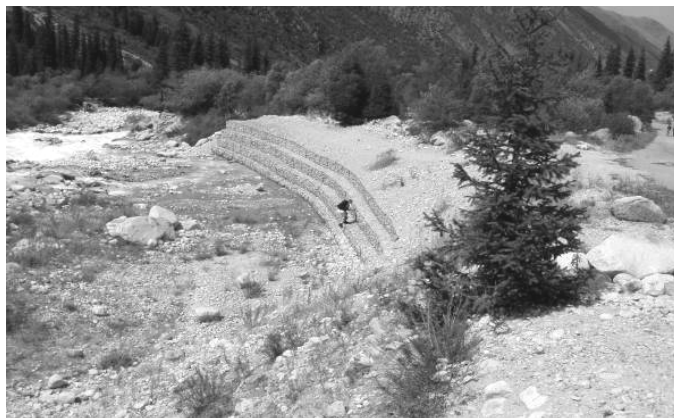
Fig. 8. Coast-protecting dam in the Alaarcha River valley
