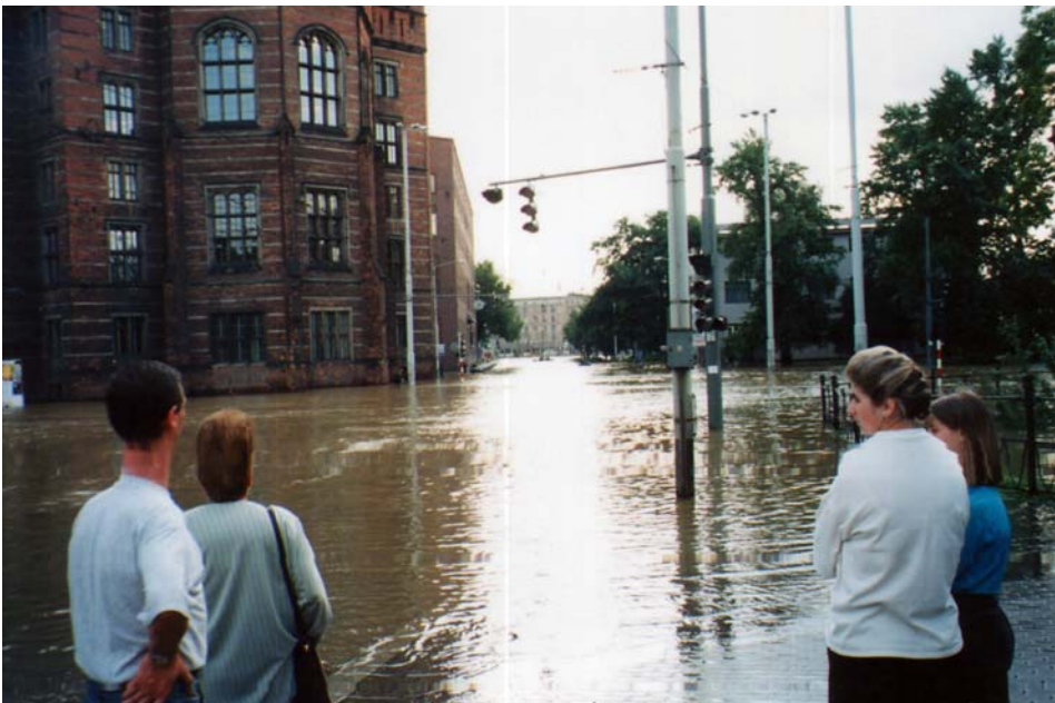
Photo 3. Court building, flood of July 1997
