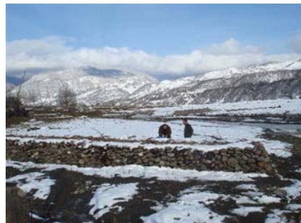
Fig.8. Gabions in Tskheniskali River, Tsageri district (March 09)
