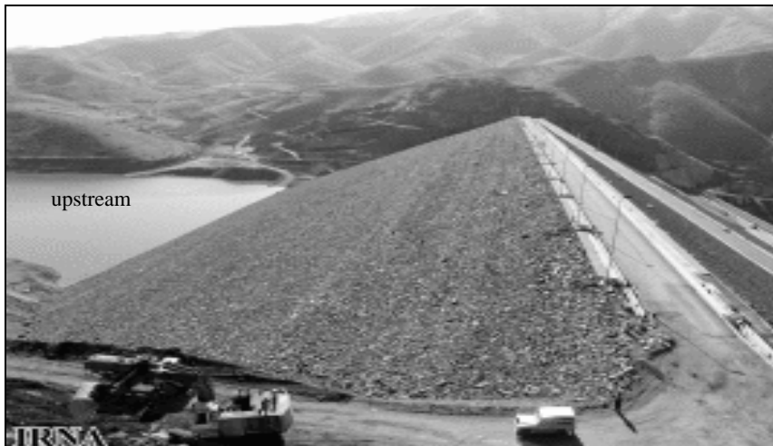
Figure 6. The site view of Ghavoshan dam body
