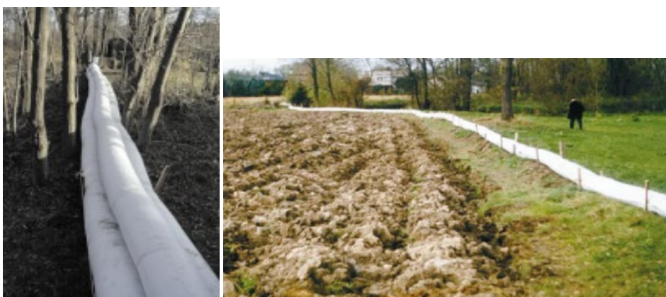
Fig. 5 Triple bag (Letohrad, Ticha Orlice River) and hose bag (Petrovice, Stonavka River)
