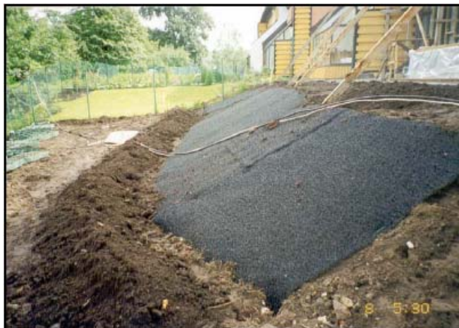
Photo 7. Mounting of “Sekumat”
