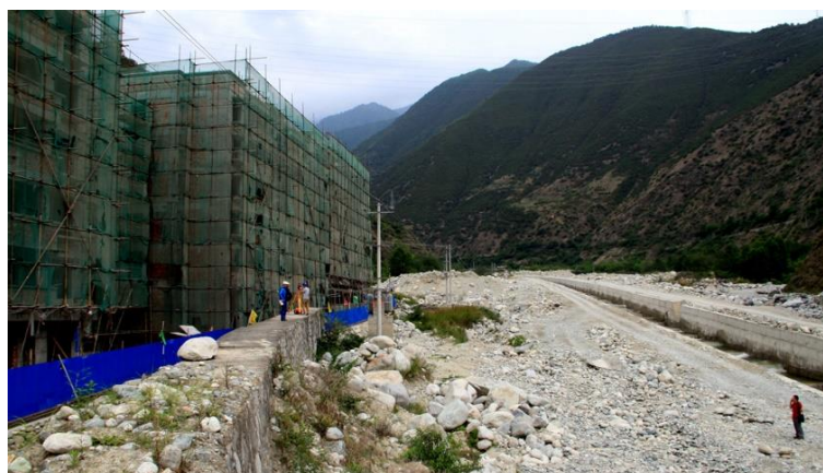
Fig. 9. Houses located on the edge of the debris flow drainage canal in the new town.
