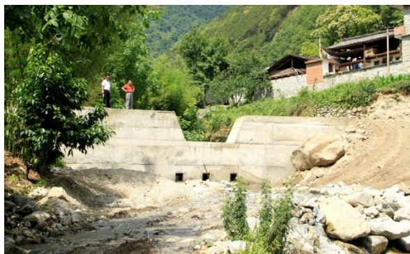
Fig. 7. Check dam in the Chejia Gully.
