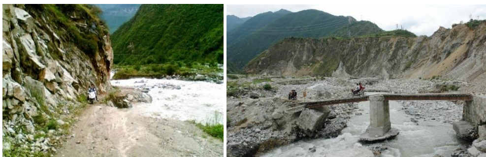
Fig. 2. (a) Debris flow destroys road; (b) debris flow destroys bridges.
