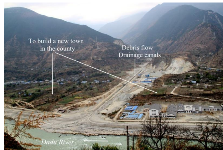
Fig. 3. Debris flow depositional fans and drainage canals in the Mohe Gully.
