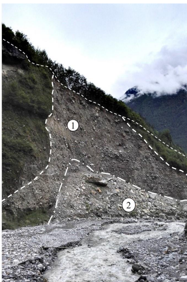
Fig. 6. Avalanche source. ①Back wall of landslide, ②Avalanche Source.
