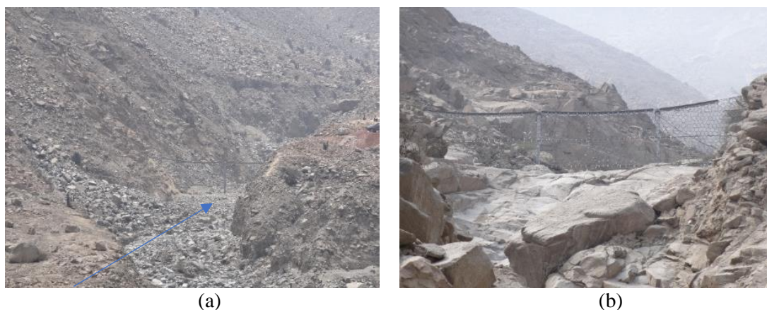
Fig. 10: two examples to illustrate the blending in of the flexible ring net barriers into the landscape making them almost invisible (blue arrow indicates barrier on the left)
