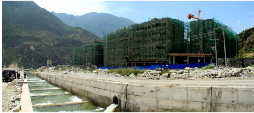
Fig. 10. Drainage canals and rib ridges.
