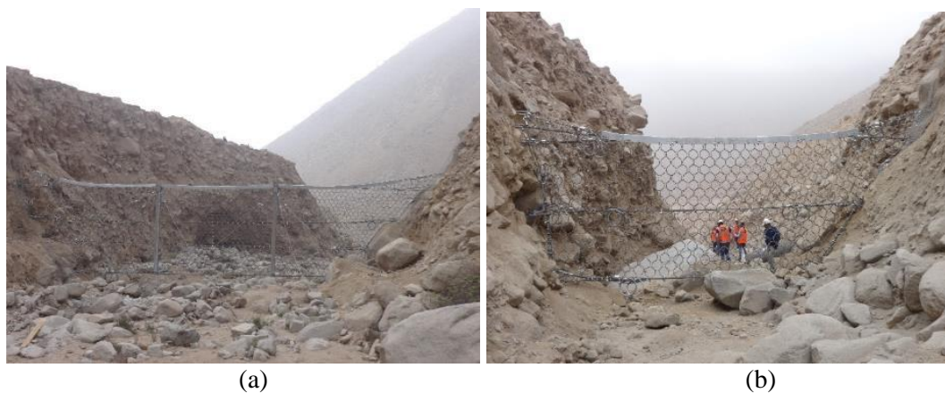
Fig. 7. UX- barriers with two posts in the channel bed (a) and VX barrier in a narrower channel (b)
