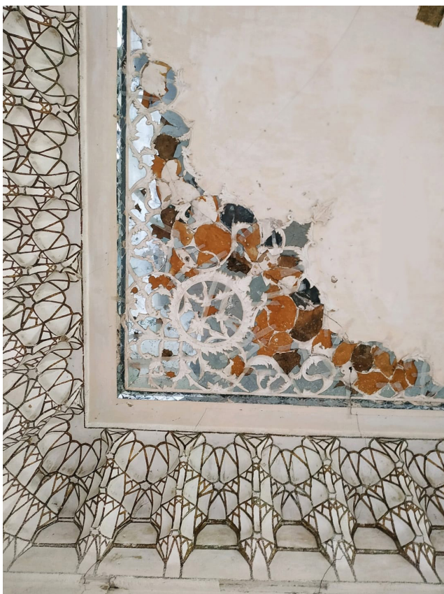
Fig. 5, 6, 7. The estate of A. Tarkhan-Mouravi. The large living room, where the stage used to be. Decorating with mirror mosaics (the base of the chandelier and at the corners of the room), decorative plaster stucco moulding in the form of stalactite ornaments of the transition from the walls to the ceiling. The works performed by the crew of Persian masters based on Chinese motives. The great hall was decorated with French wallpaper. The period between 1821 and 1831. Photos from the archive of Ludmila Narikaeva.
