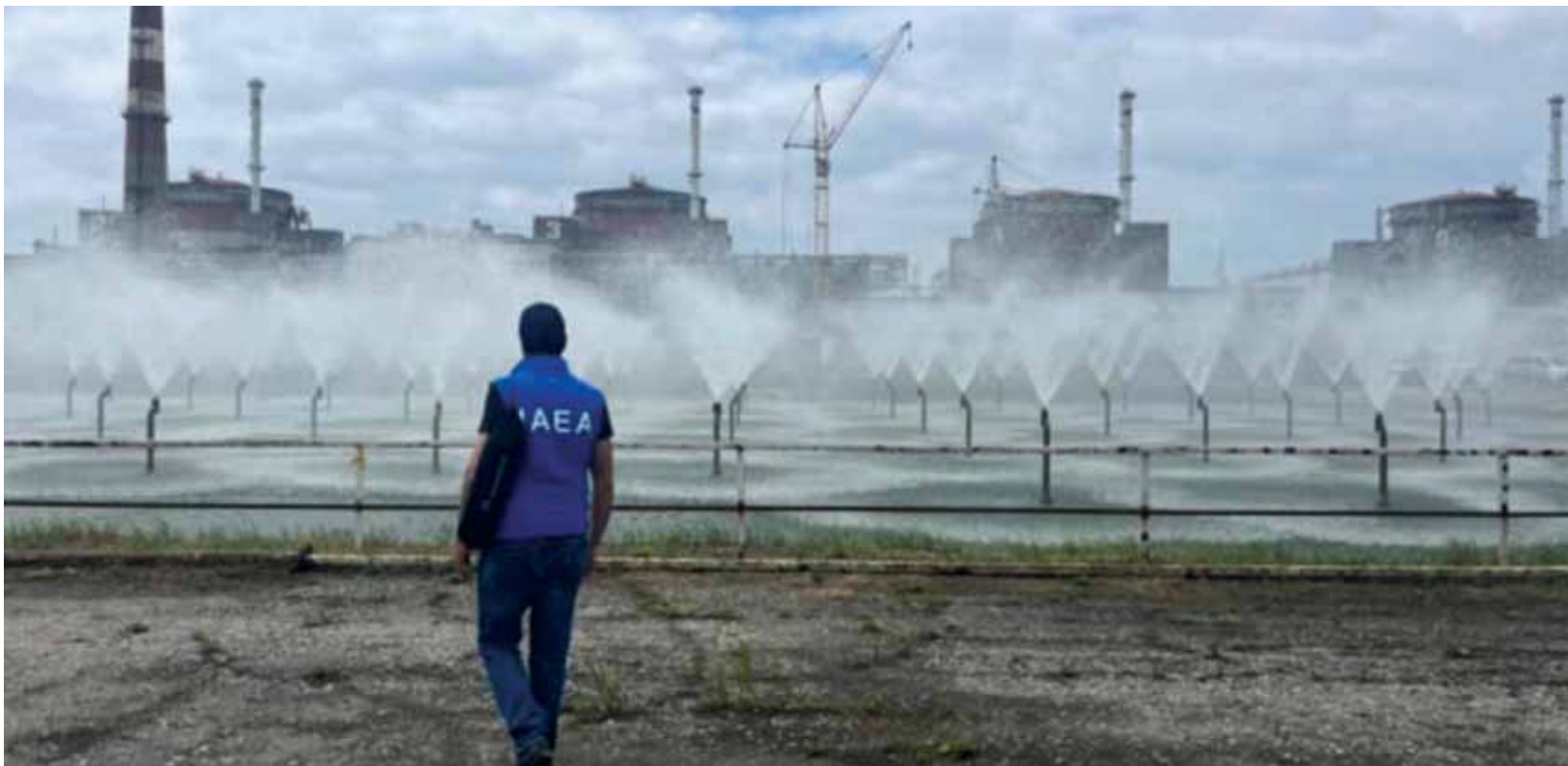
Zaporizhzhia Nuclear Power Plant during the visit of the International Atomic Energy Agency expert mission in 2023. Source: IAEA via Reuters
